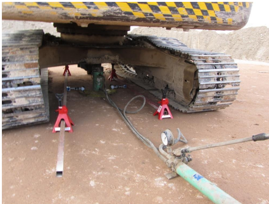
Plate (2): Plate Bearing Test for Location of Tank HFO Set 6
