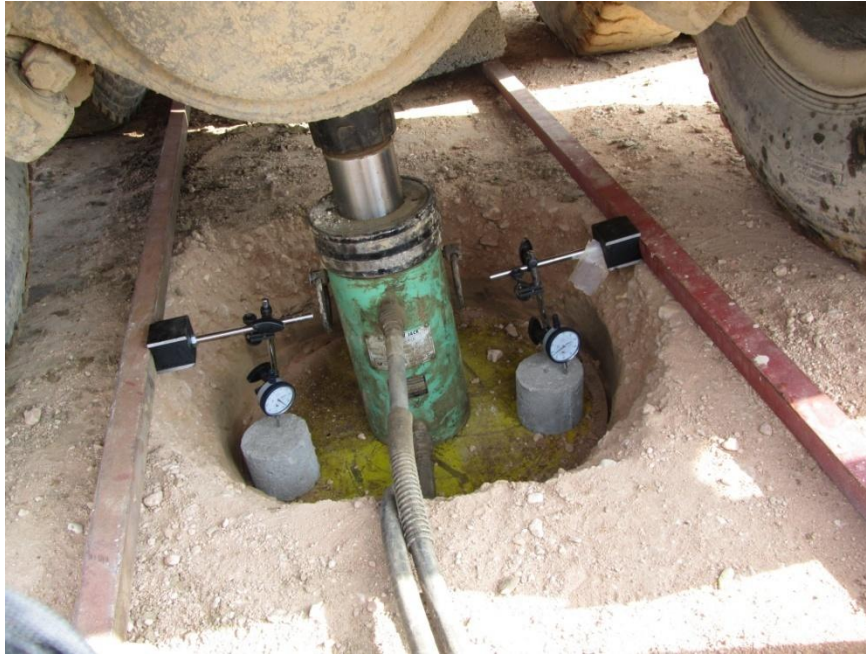
Plate (1): Plate Bearing Test for Location of Tank HFO Set 5
